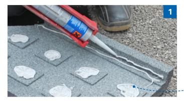
• The glue is laid on in circular form on the outstanding squares and along the rounded edge.
