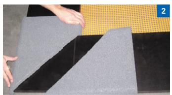
• Place the impact protection tile flush on the frame and tap strongly.
